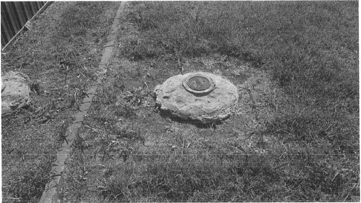
Photograph 6: Sewer point running along west boundary.
