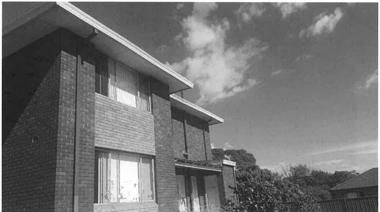
Photograph 5: Paint flaking – Based on age potential lead. Potential ACM in roof eave.
